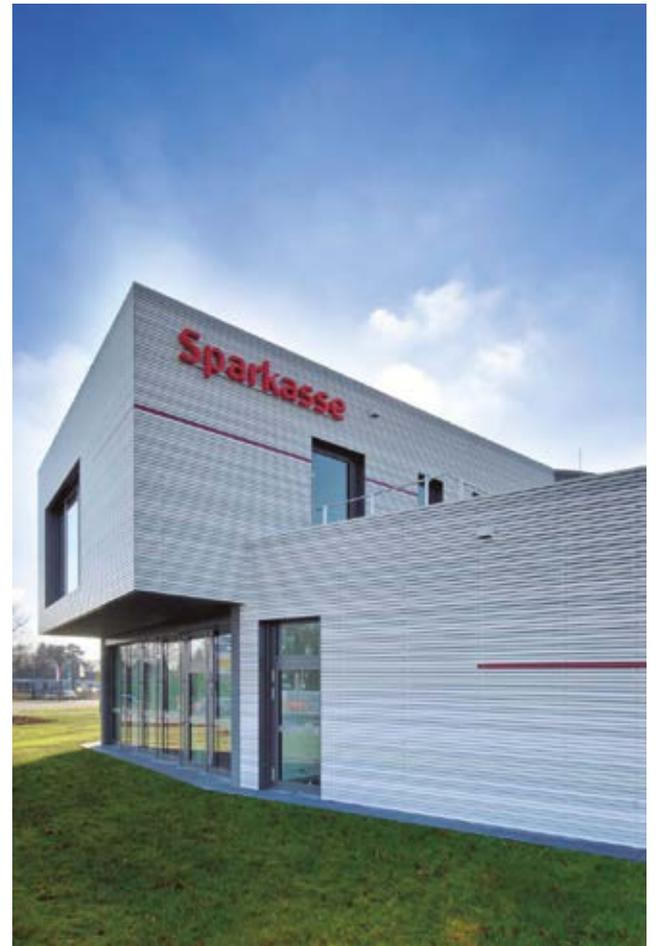
The rear-ventilated facade of Fshape is available in a variety of color design options. With this aluminum façade system, façades can be realized in simple gray tones as well as stronger colored accents. This lamella facade always emphasizes the cubature of the building. Both the protrusion as well as the recesses convince through the great plasticity and purity of the form.
