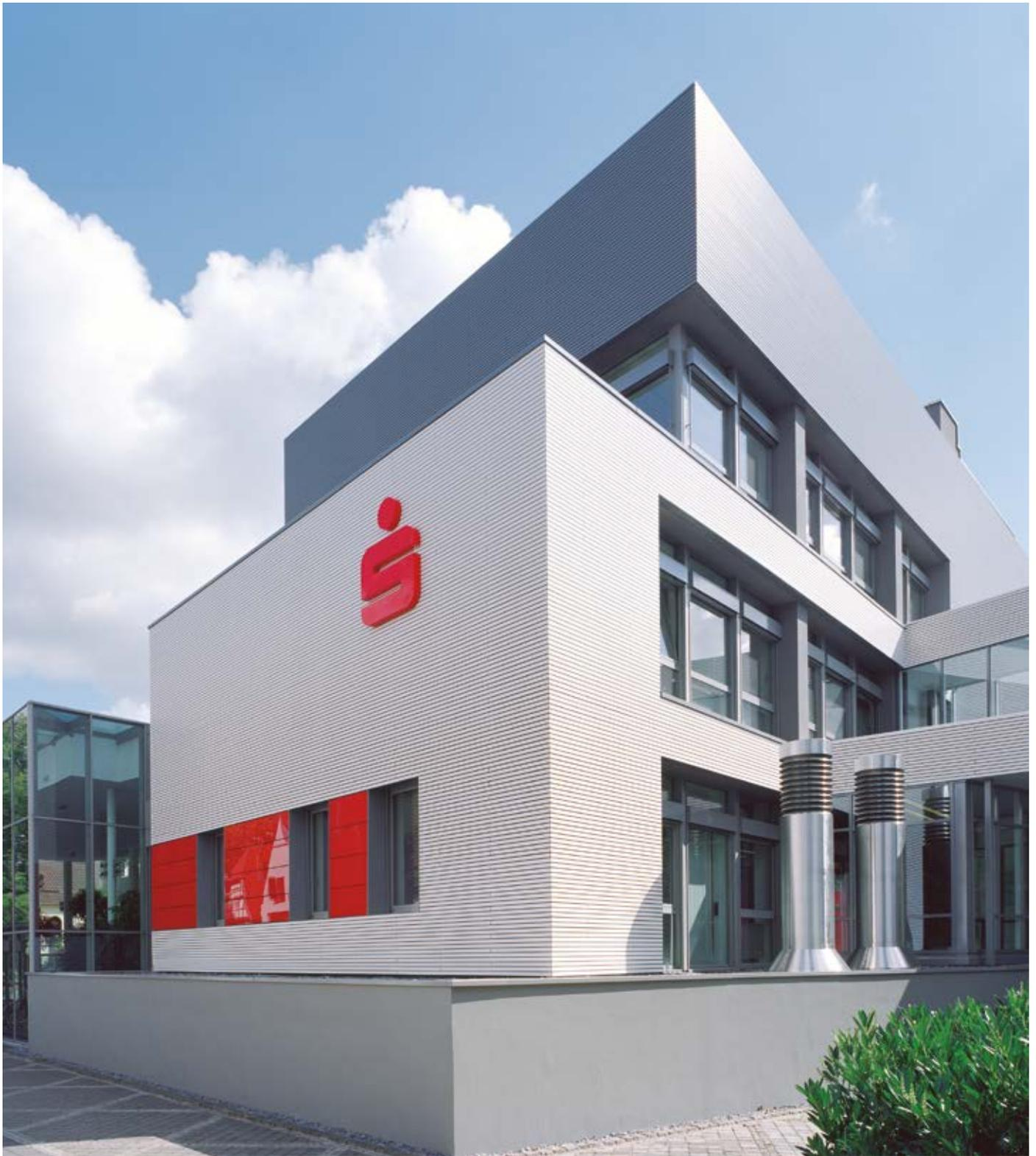
The Sparkasse in Rheda-Wiedenbrück is a good example of the high plasticity of the building elements, which is enabled by the Fshape aluminum façade system. This façade convinces with its extremely clean building edges. This is particularly apparent in the case of the building openings that spring inward. At the same time, this
