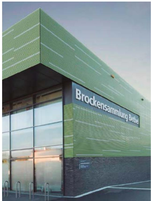
This building is an example of what makes the Fshape aluminum facade system so special: the façade of aluminum lamellas enhances the building cubature and inspires by a very great optical purity. At the same time, the lamellar façade allows for a very lively facade picture due to different tones in the planking.
